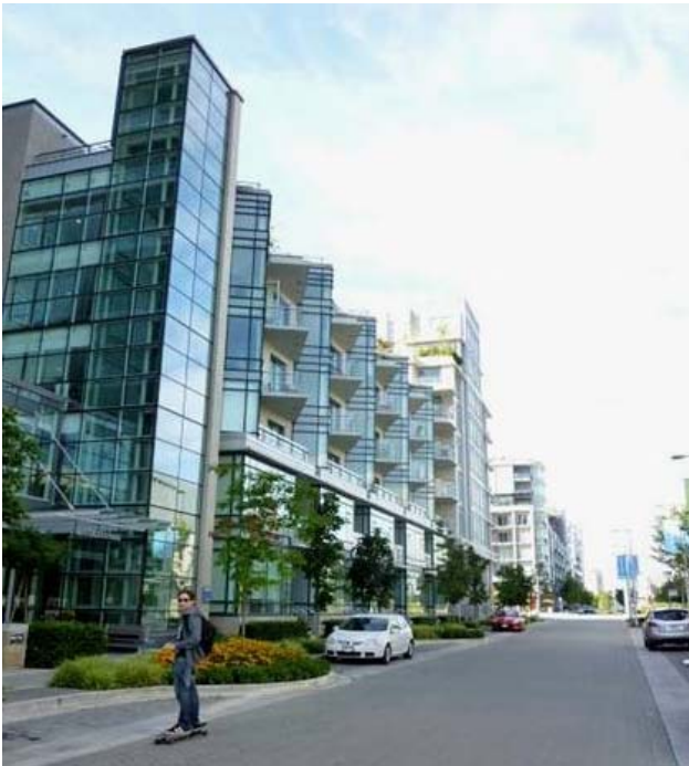
Figure 2: Buildings on 'A' Streets are continuous along the length of development blocks and integrate seamlessly with the public realm to produce lively, animated, pedestrian oriented frontages.
